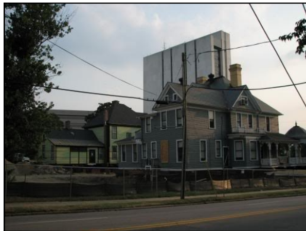
The Jordan House in 2008 prepped to be moved to its current location on the corner of Peace and Blount.
